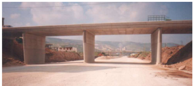
Construction Of Over Pass Bridge
