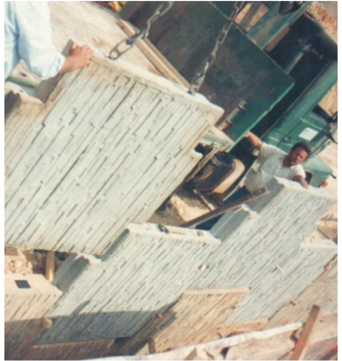
Installation Of Reinforced Earth Wall Panels
