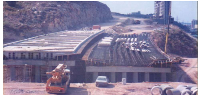
Construction Of Bridge Deck
