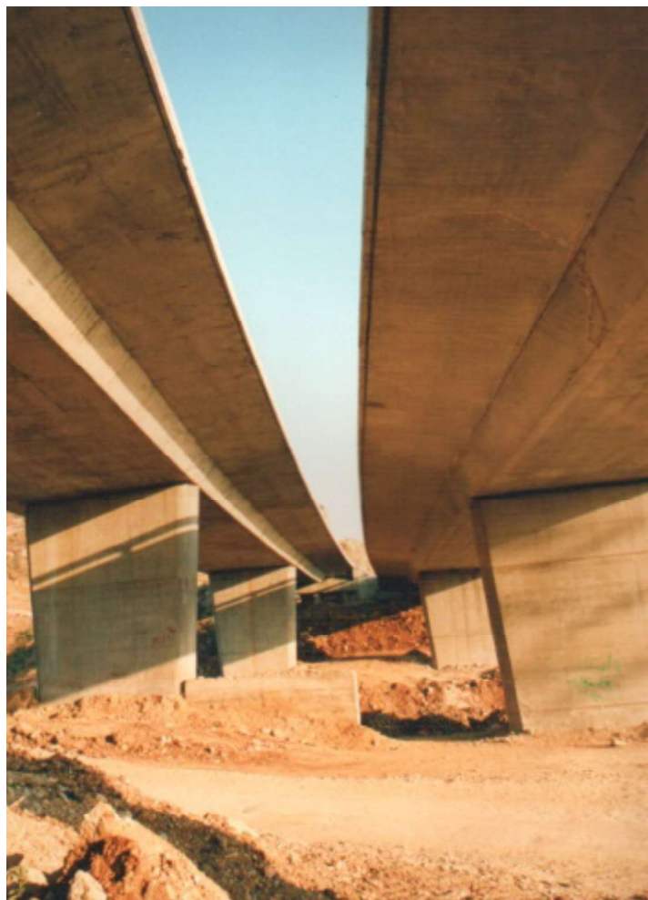
Over Pass Bridge
