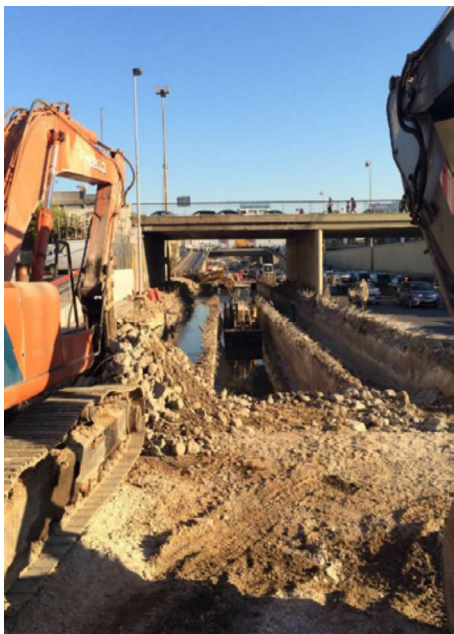
Demolition of existing box culvert
