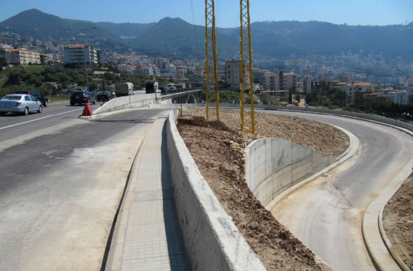
Prime Coat Prior To Asphalt Binder Course Paving
