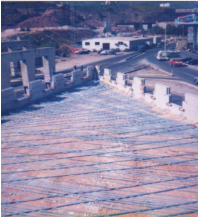
Construction of Reinforced Earth Wall
