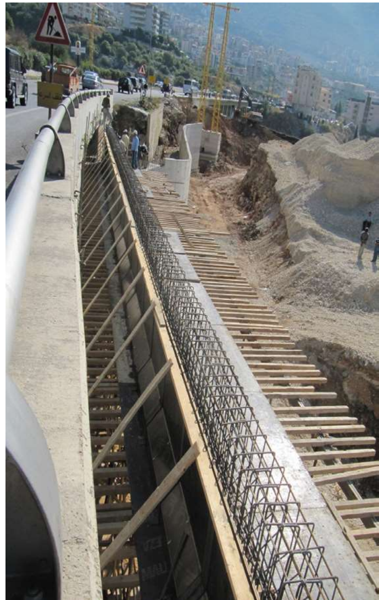
Girder Beam-Installation
