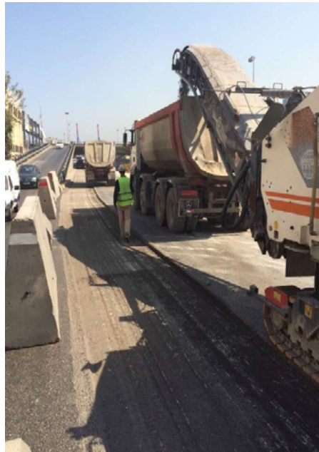
Asphalt-milling
