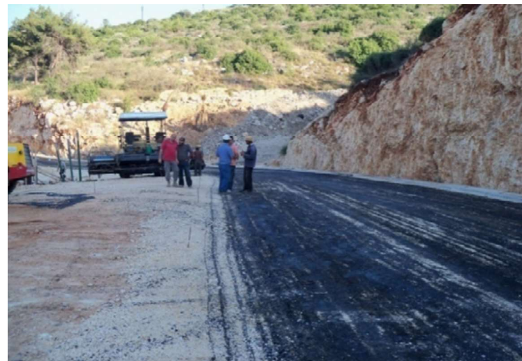
Prime Coat Prior To Asphalt Binder Course Paving
