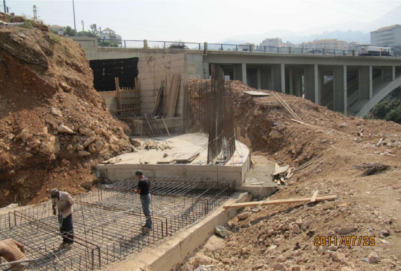
Retaining Walls Foundations
