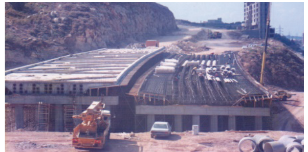
Construction Of Bridge Deck
