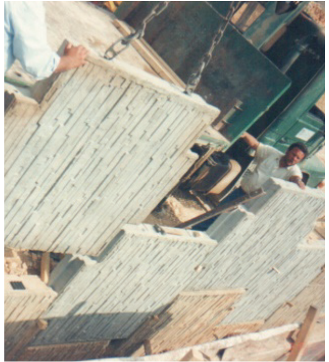
Installation Of Reinforced Earth Wall Panels
