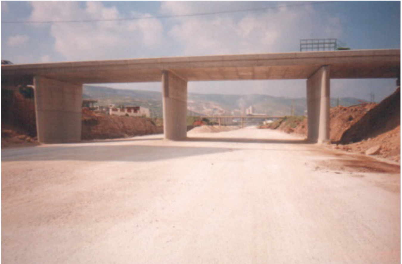
Construction of Over Pass Bridge
