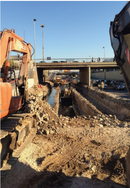
Demolition of existing box culvert
