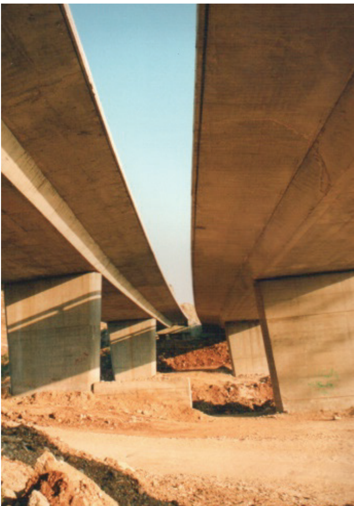
Over Pass Bridge
