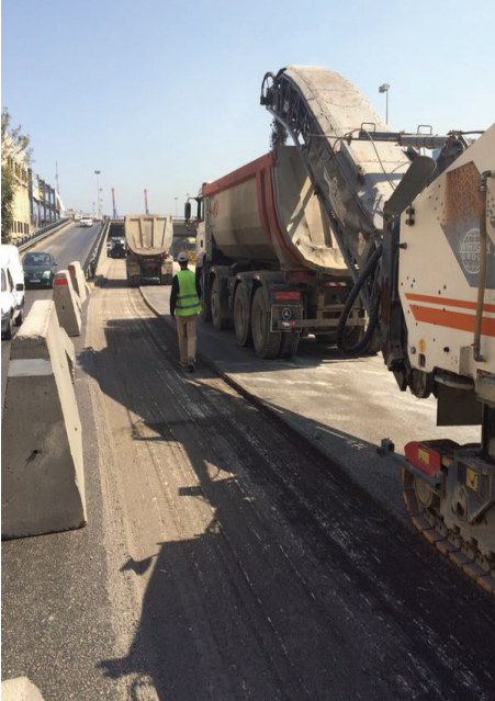
Asphalt-milling
