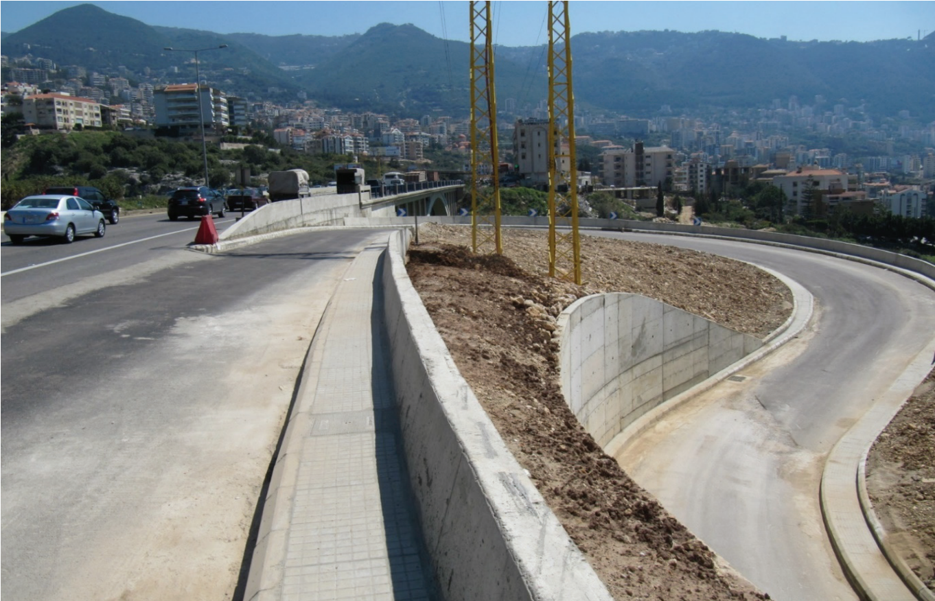
Prime Coat Prior To Asphalt Binder Course Paving
