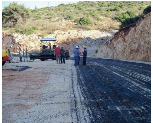
Prime Coat Prior To Asphalt Binder Course Paving
