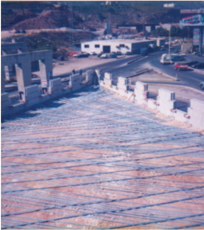
Construction of Reinforced Earth Wall
