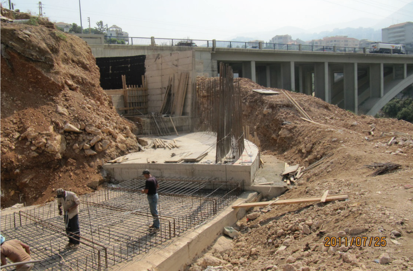
Retaining Walls Foundations
