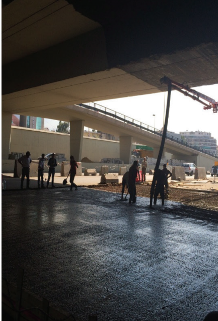
Concreting of boxculvert top slab
