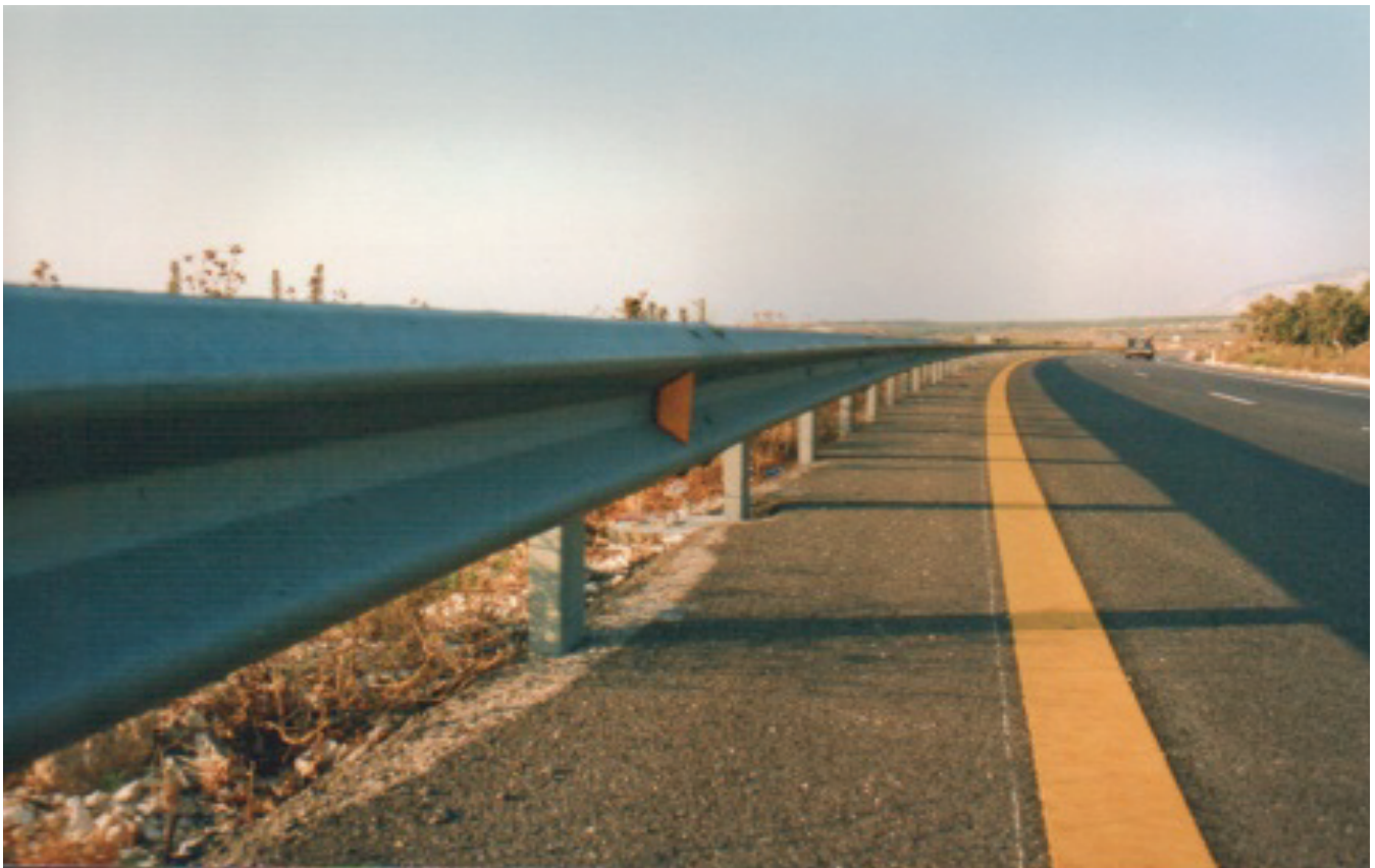
Road final shape - Steel guard rail - Wearing course - Edge marking yellow line
