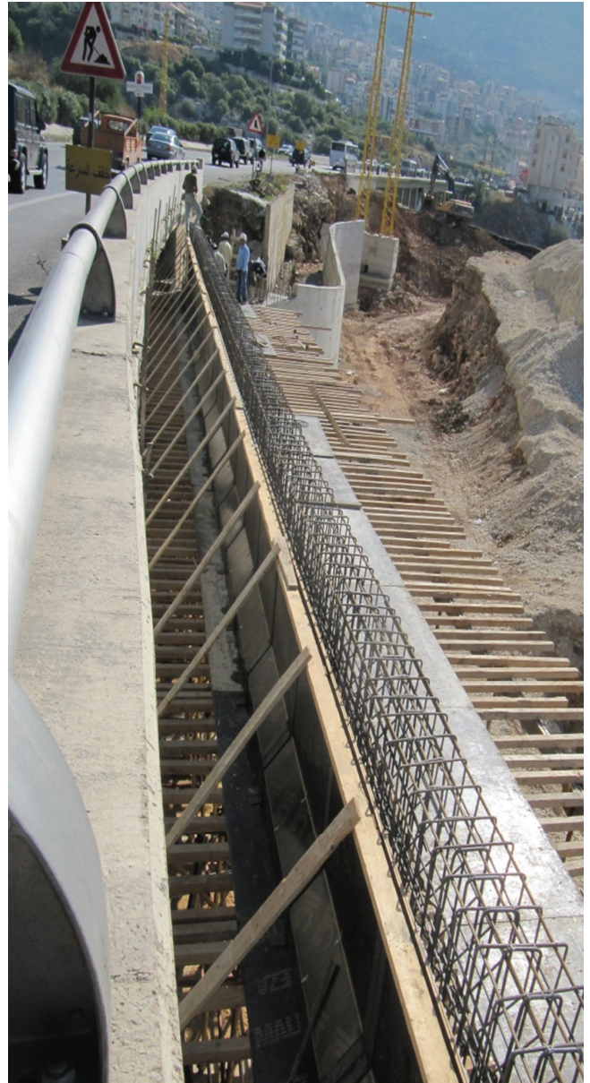
Girder Beam-Installation
